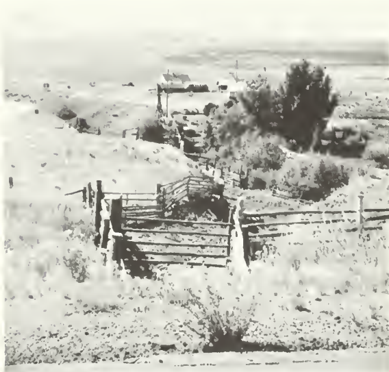
Looking North from NORTH ENTRANCE
